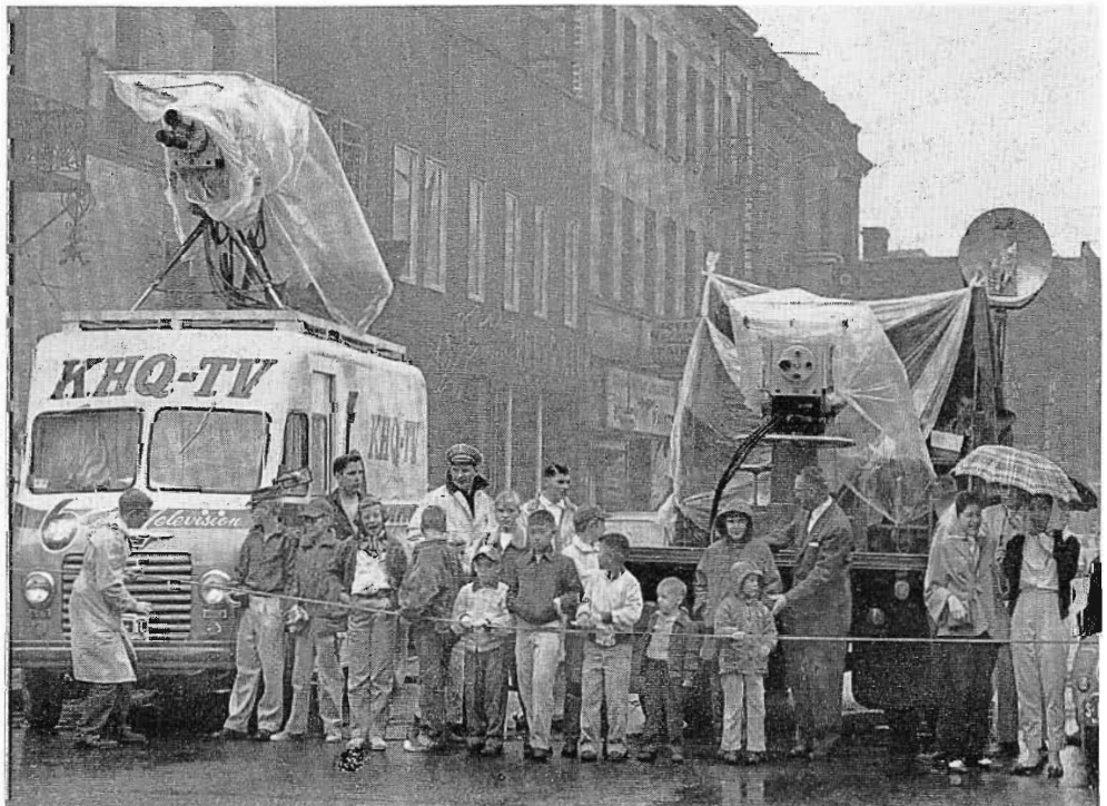
FIG. 5. KHQ-TV used its own color mobile unit and a rented flat-bed truck to cover the parade. Note also microphone with parabolic reflector (right) to pick up music and crowd noise.
