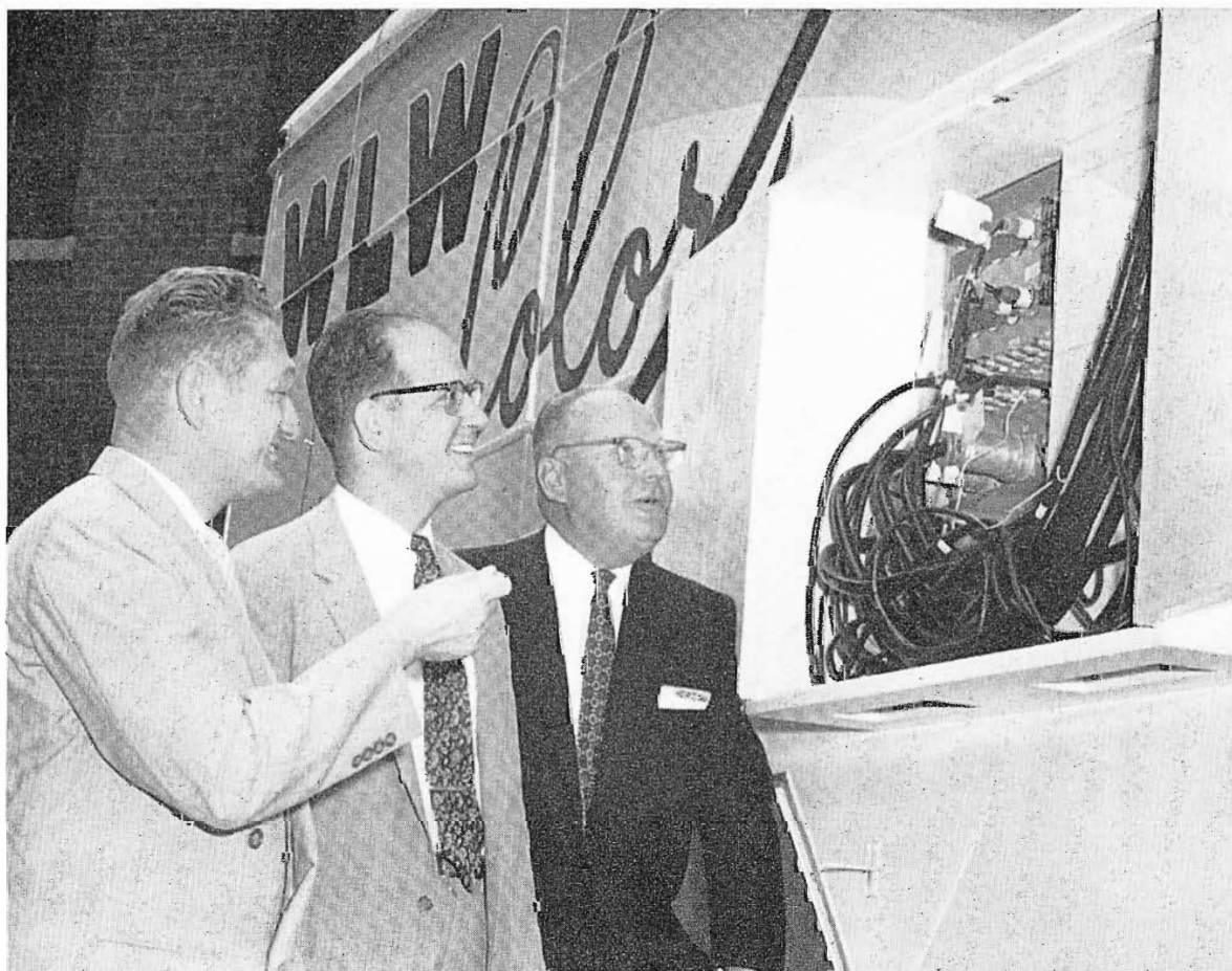
FIG. 8. Located on the side wall of the mobile unit are connectors needed to integrate mobile control room with existing control facilities.
